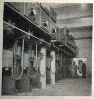
IN MODERN GREECE we have constructed a considerable amount of switch gear, of which this switchboard, in an Athens sub-station, is a good example. It comprises metalclad switchgear operating at 22,000 volts, and is part of the large expansion of electricity supply now being carried out in that country.
